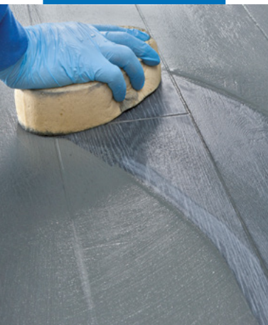
Cleaning and finishing the joints with a hard cellulose sponge
