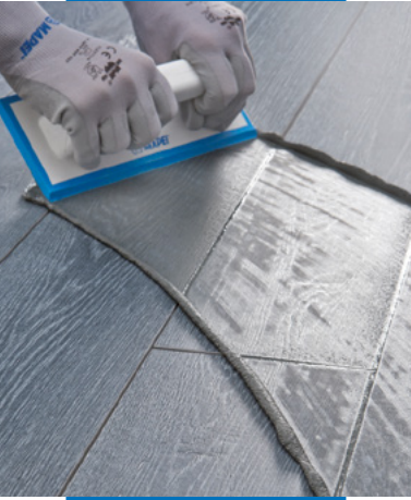
Spreading Ultracolor Plus on wood-effect porcelain floor tiles with a rubber float
