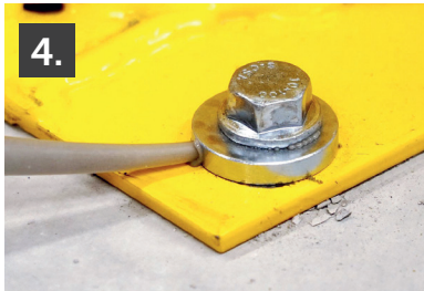
4.) Fill the annular gap between Concrete screw and fixture through the hole of the Filling Washer until resin leaks out of this hole.
