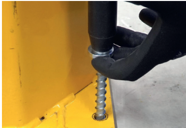
2.) Drive in concrete screw with filling washer until the anchorage depth h_{nom} is reached
